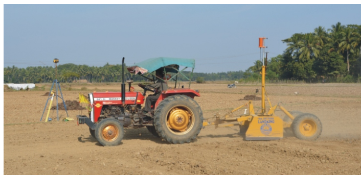
Land leveling using laser guidance
